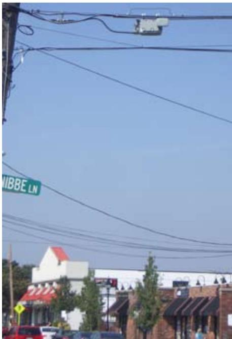
**Figure 4. BelAir I00S deployed on aerial strand.**
