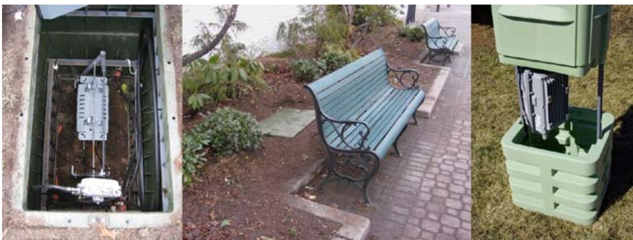
**Figure 5. BelAir 100S vault and pedestal installations.**
